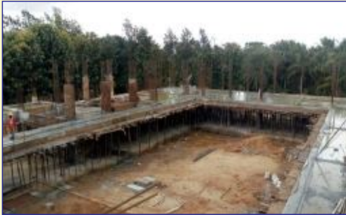
Boys hostel ground floor roof casted.Ladies hostel ground floor in progress.
